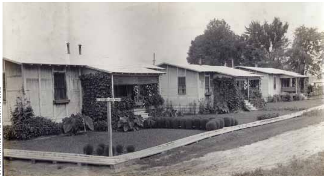
At the beginning of World War I, DuPont built villages for employees of its gun cotton factory in Hopewell. The villages included paved streets, schools, churches and shops.
